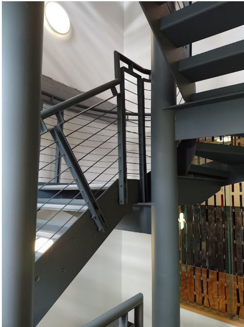
View of one of the metal stairways.
