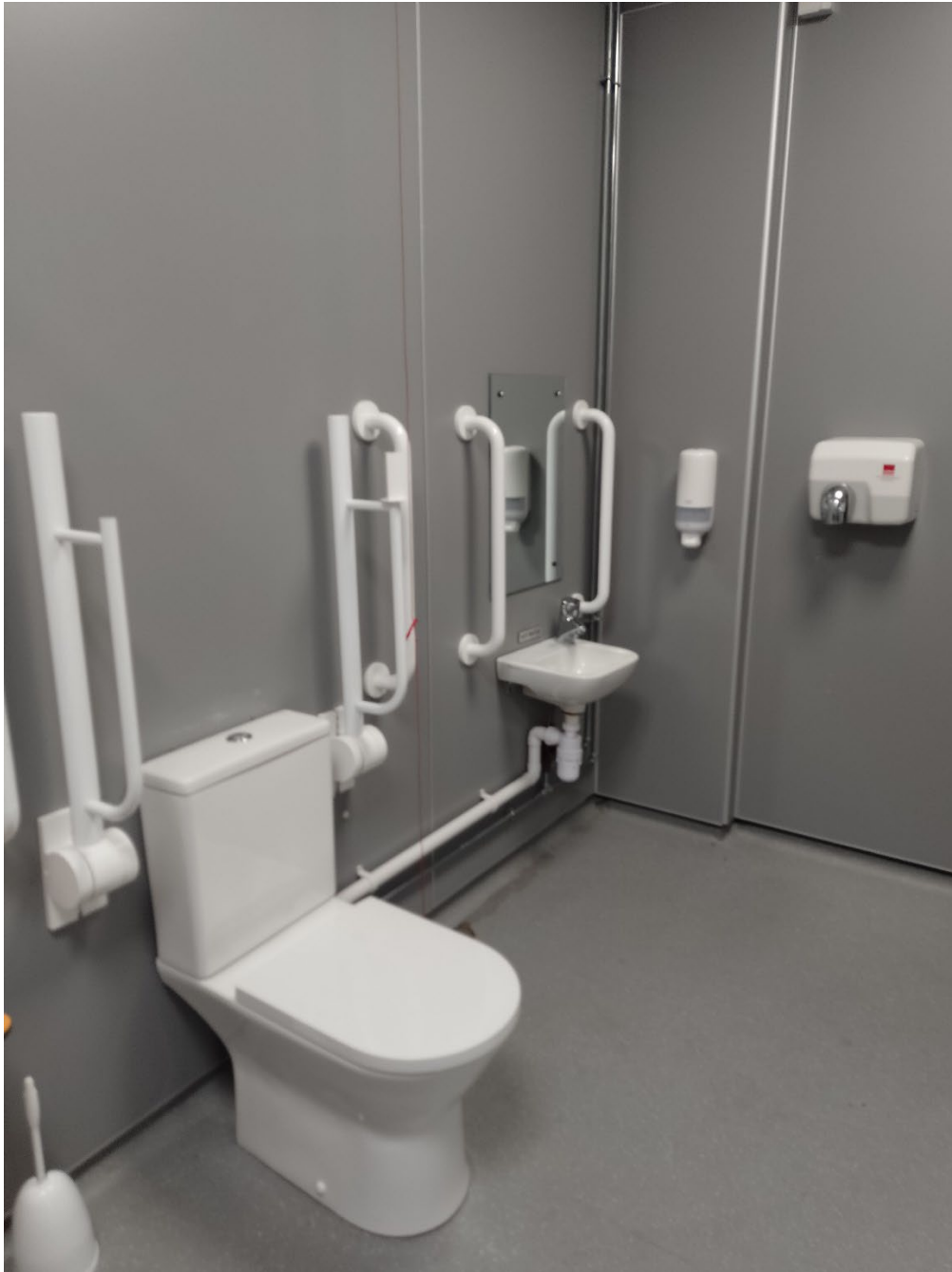
Accessible changing room toilet with grab rails
