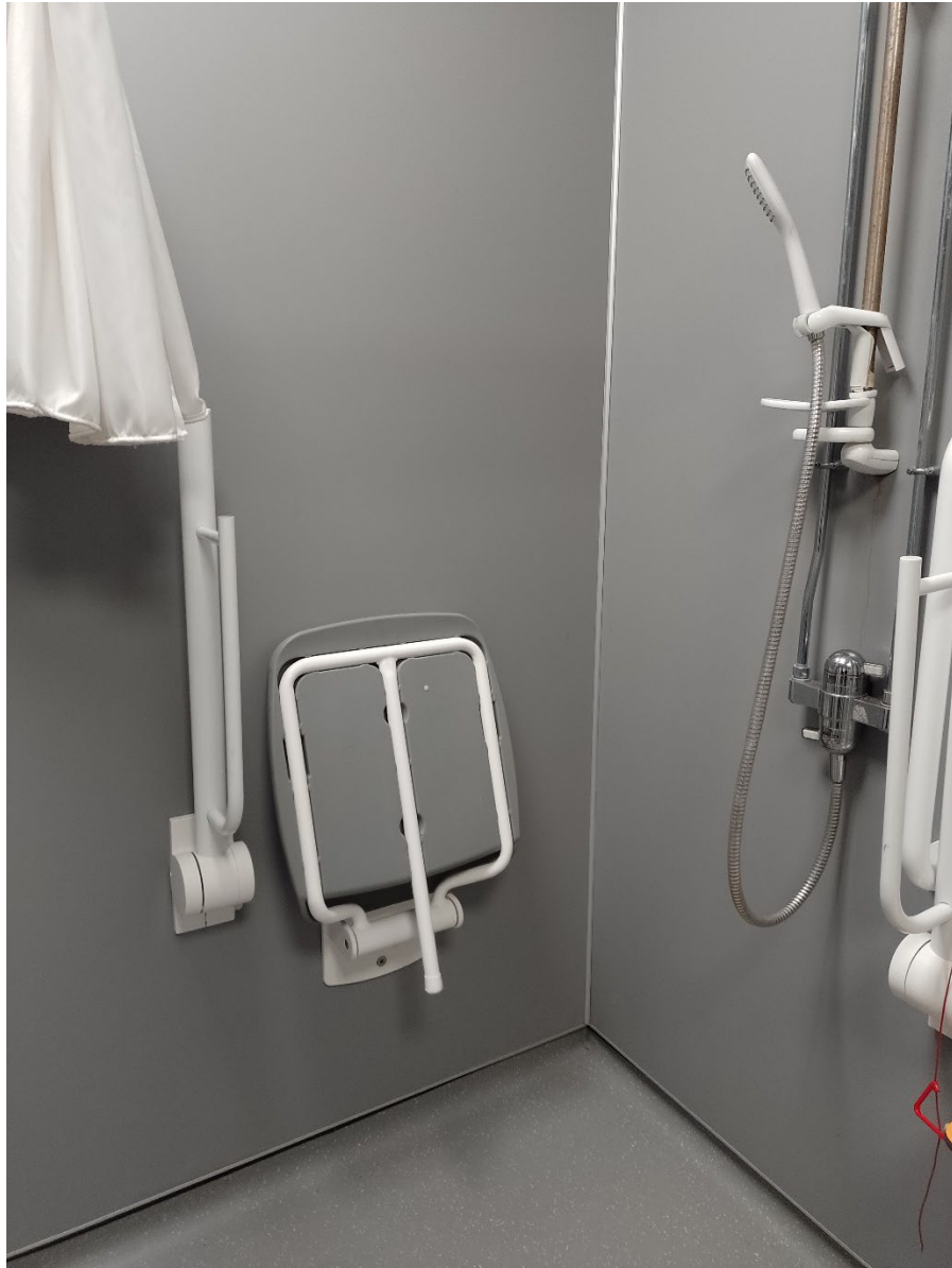
Shower with fold down seat, grab rail and alarm in the accessible changing area
