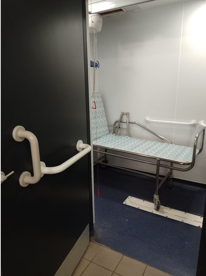
Accessible changing room with hoist and changing bed.
