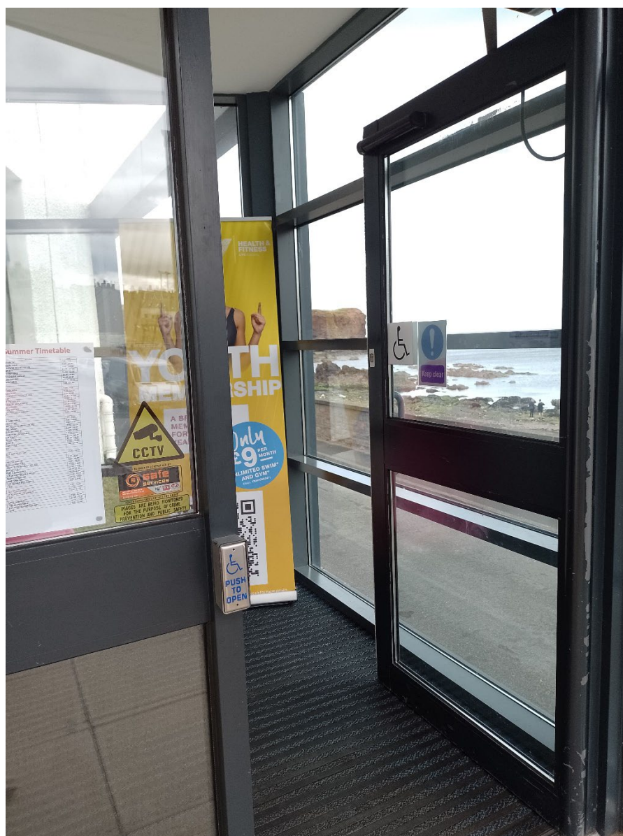
View of push button main door
