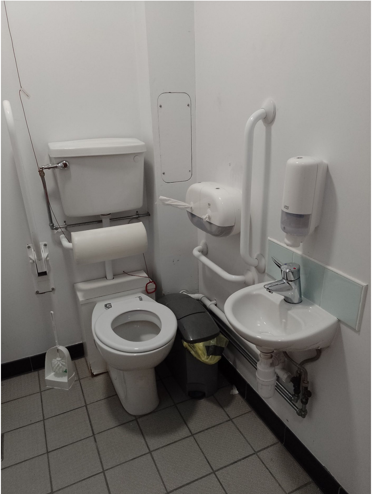
Toilet with grab rails, low level basin, adequate floor space for maneuvering.
