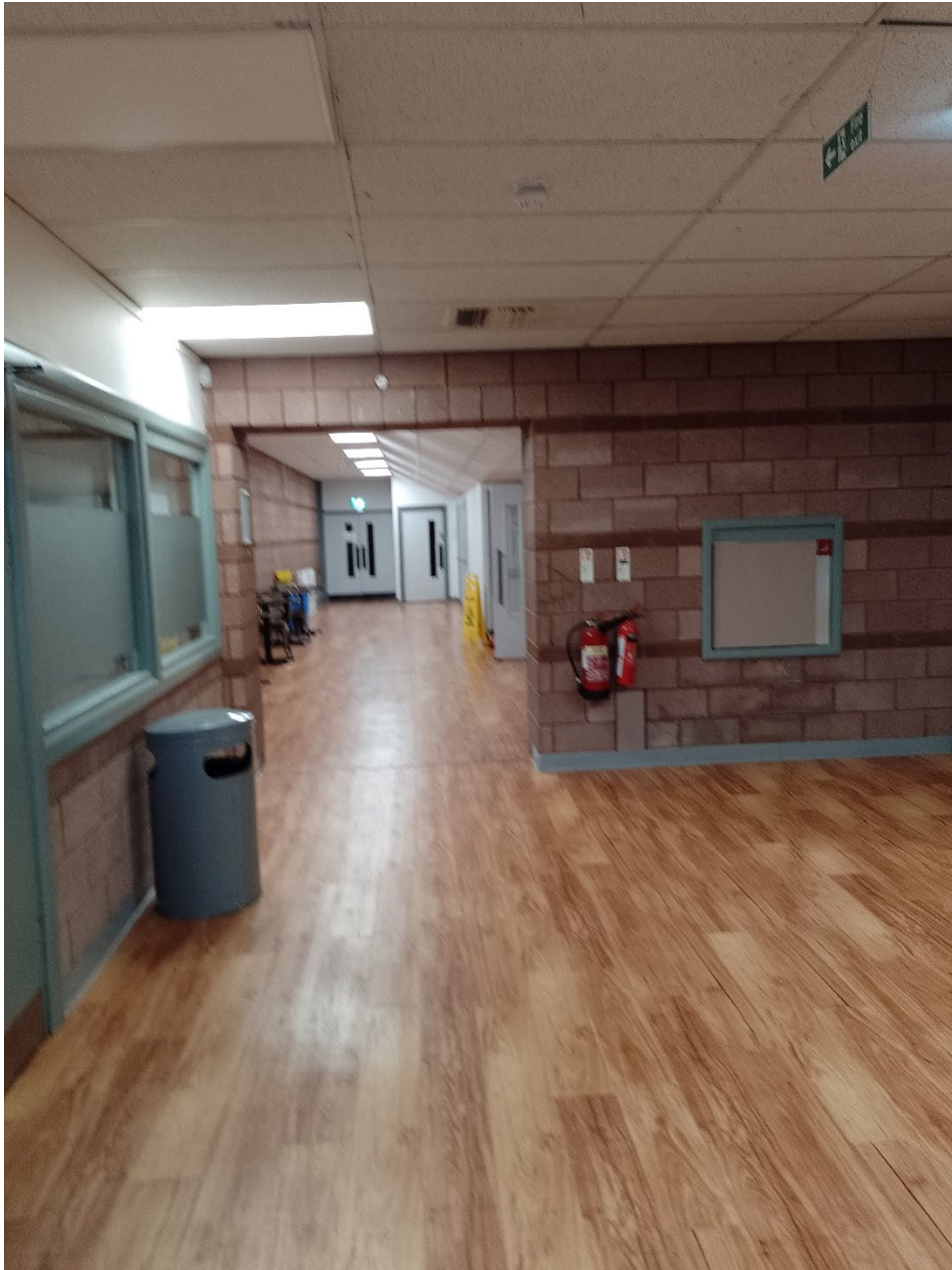
Corridors are wide with smooth laminated flooring.
