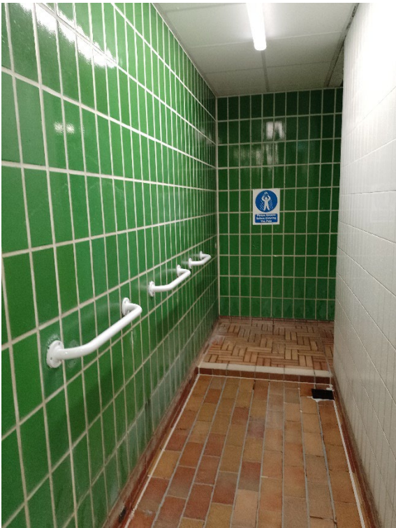
Foot bath and access to main pool
