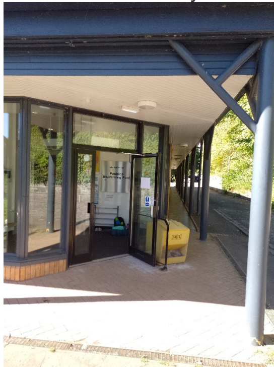
View of push button main door and the covered approach route
