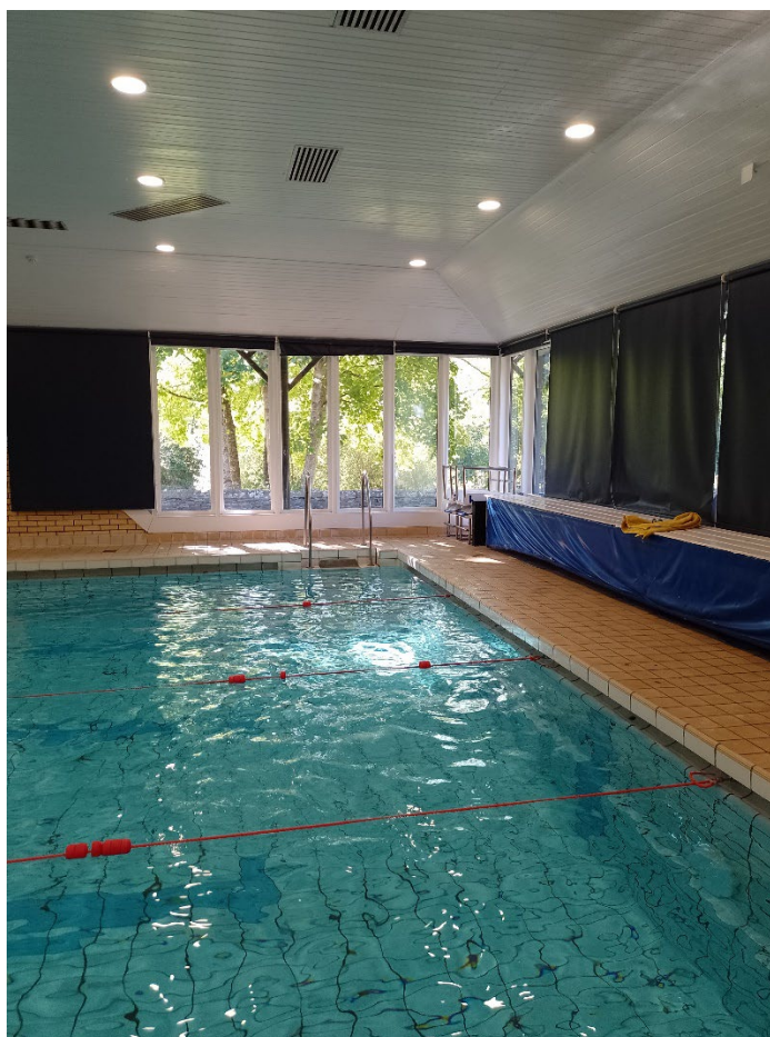
The pool hall has large windows at either end, these may be covered with blinds when it is sunny.
